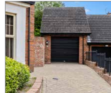
GARAGE: 21' 4" x 10' 4" (6.51m x 3.14m) Power and light, roller shutter door
