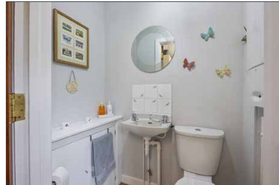
WC: White suite comprising: wall mounted wash hand basin, push button WC, Worcester gas boiler.
